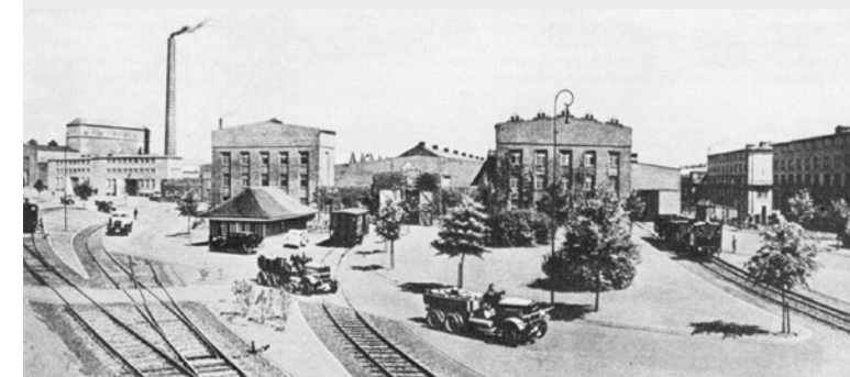
Contemporary photograph of the Henschel factory buildings
